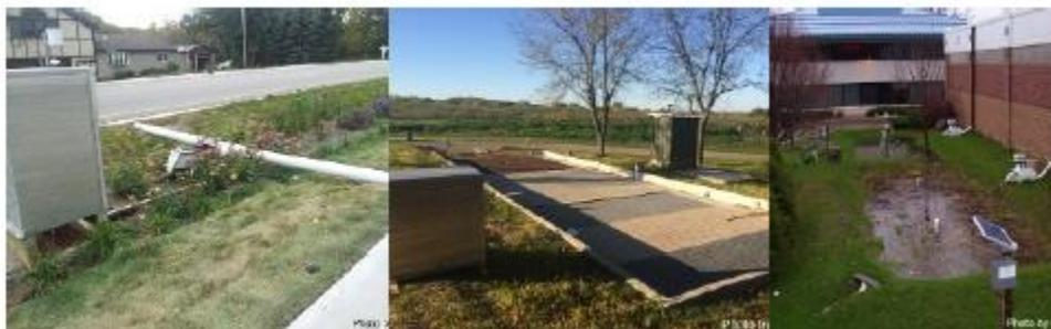
**Figure 2. Bioswales, permeable pavement, and rain garden (courtesy of USGS).**
