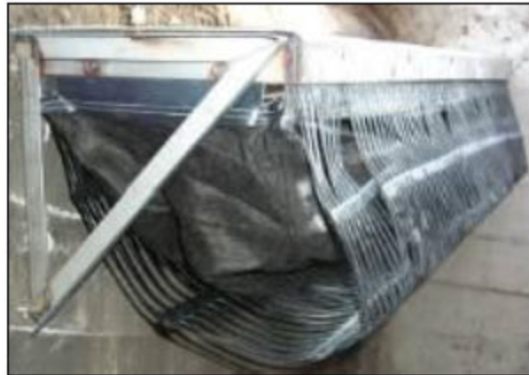
Figura 6-4 United Store Water Drainpac Curb Inlet 17
