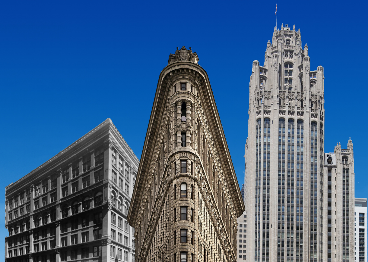
Home Insurance Building Chicago 1885
